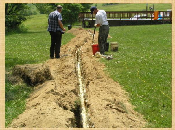
Subsidence cracks over coal mine, cleaned out and foamed WV DEQ photo
